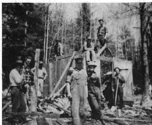
MEMBERS AT CANONTO HOLD "BEE" TO BUILD KITCHEN ON CHURCH.
