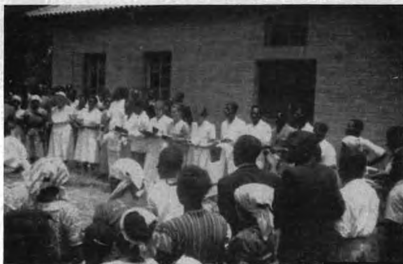
DEDICATING NEW WARD BUILDING AT CAMUNDONGO Angola
