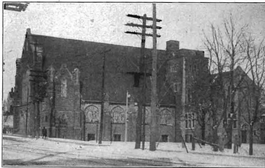
YONGE STREET METHODIST CHURCH, TORONTO Burke, Horwood & White, Architects.
